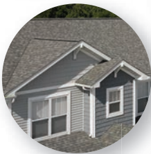
Roofing and Ventilation
